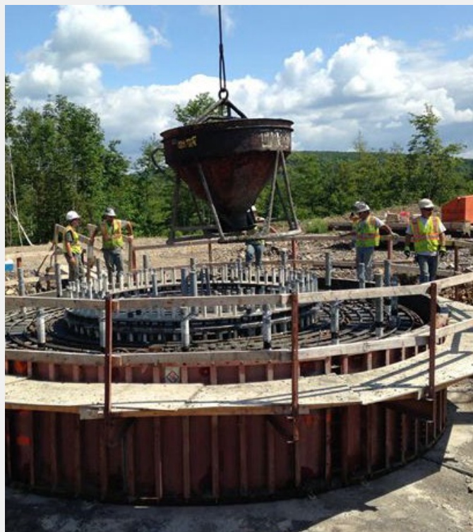
Construction workers installing the foundation of one of the V-112 Vestas turbines at the Oakfield wind project in Aroostook County, ME.
